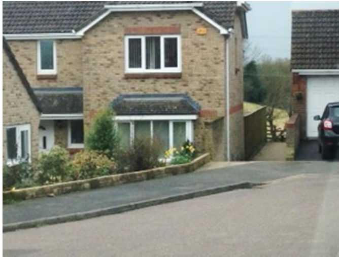
Taken from Claremont Field looking west at a potential pedestrian access between existing houses
